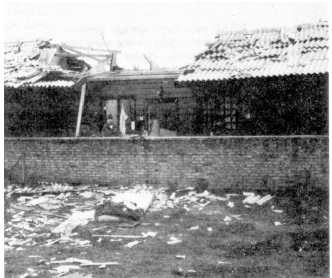
Brick revetments constructed about billets at Pleiku Air Base to protect against shell fragments. Such revetments were useless against direct hits
